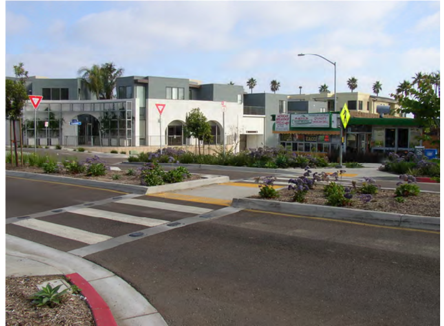
Mid-block crosswalks with pedestrian refuges can help increase pedestrian connectivity while allow pedestrians to cross the roadway in two steps.
