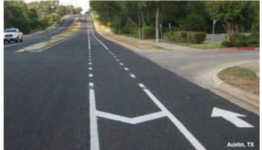
Example striping that complies with California guidance to dash buffer to indicate crossing the buffer is allowed for turning or parking maneuvers. Image source: Fehr & Peers. San Jose, California (2012).
