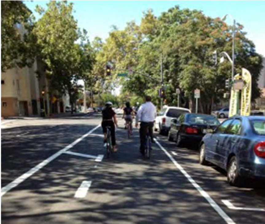
Example buffered bike lane with chevron-style buffer zone, which breaks at intersections to denote vehicle crossing locations. Image source: NACTO. Austin, TX.
