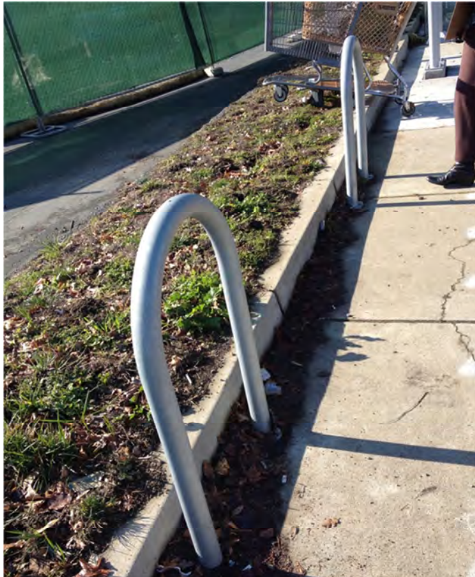
Bike racks must be placed so that both sides are accessible for use; this photo illustrates poor rack placement.
