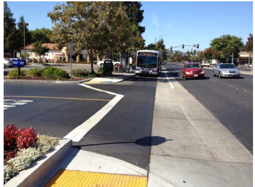
Example of a discontinuity in the sidewalk on Dublin Boulevard, where a bus pull-out is located.
