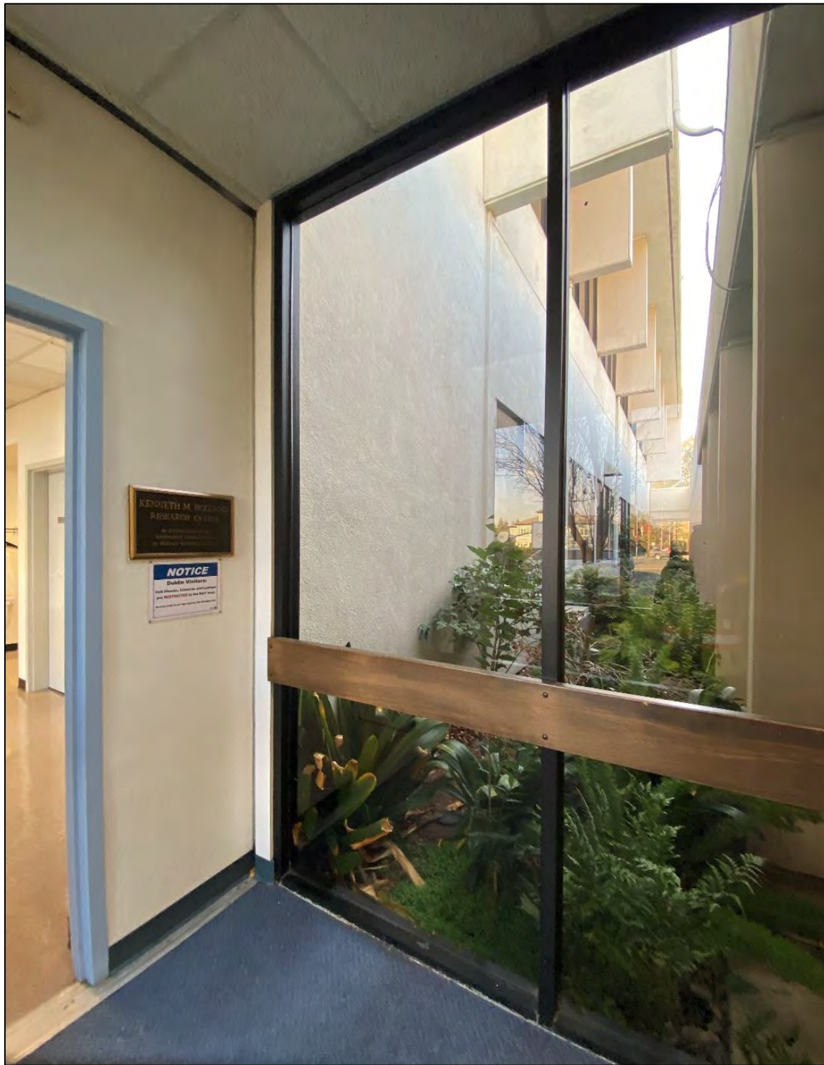
Photograph 16: Northern end of central courtyard, facing south, December 16, 2022.
