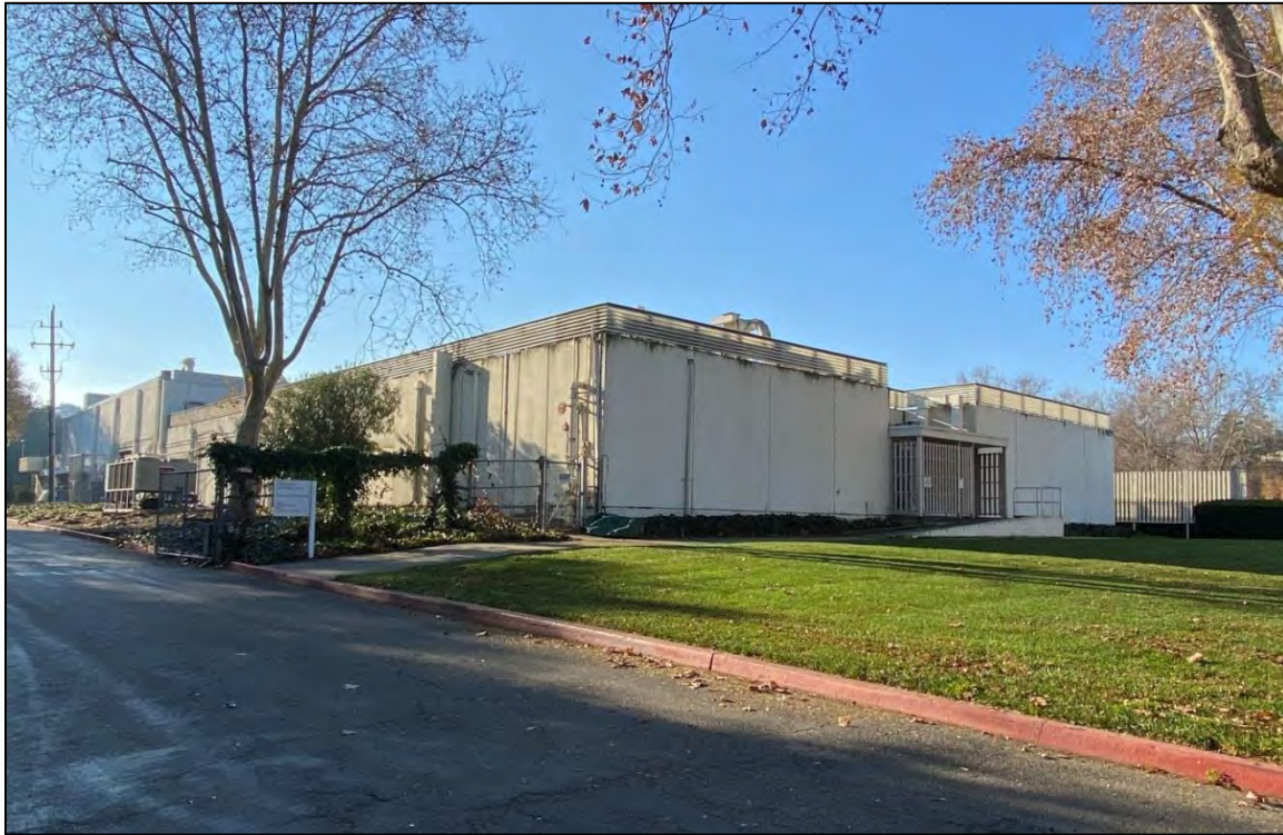
Photograph 1: Northeast corner of building complex showing the 1962-constructed portion, facing southwest, December 16, 2022. Note this is the original 1962-constructed section of the complex.
