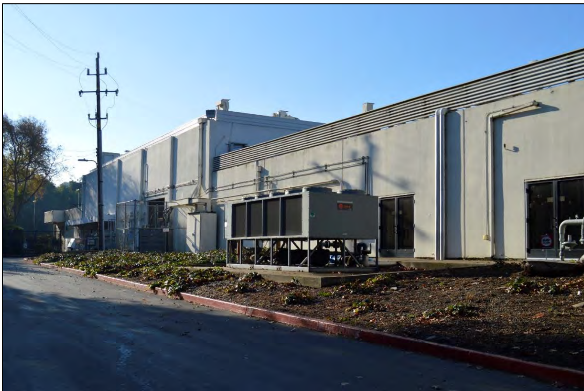
Photograph 12: North end of the east side of building complex, facing south December 16, 2022. Note most of this side consists of the original 1962-constructed section.
