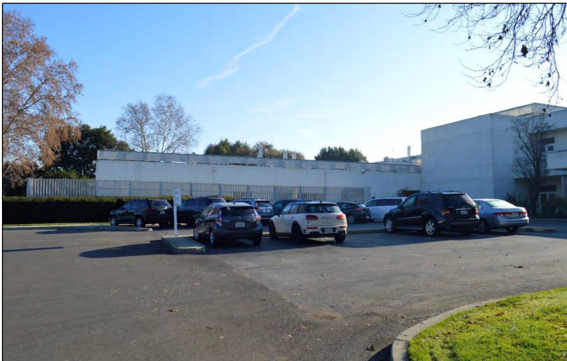
Photograph 2: West side of original 1962-construction section of the complex and primary entry on far right, facing southeast, December 16, 2022.
