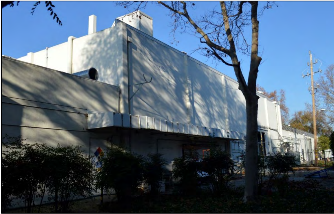
Photograph 11: South end of the east side of building complex, facing northwest, December 16, 2022. Note most of this side consists of the original 1962-constructed section.
