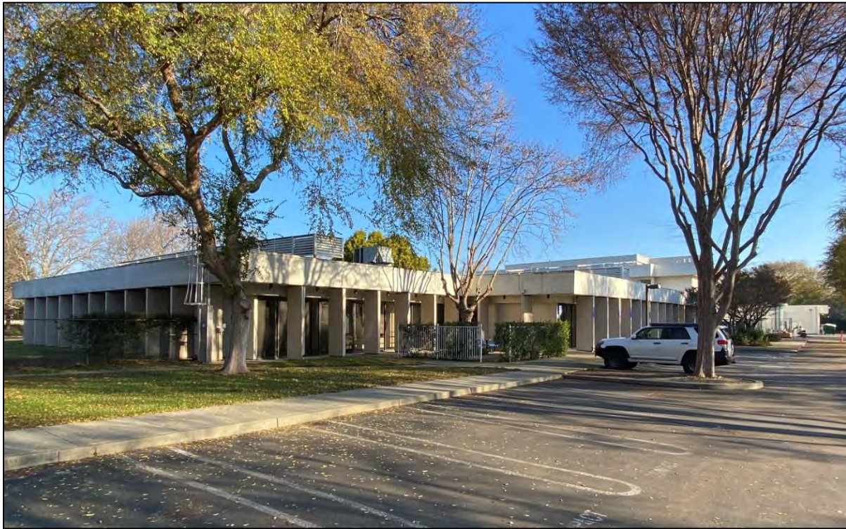
Photograph 5: Overview of west and south sides of building complex, facing northeast, December 16, 2022.
