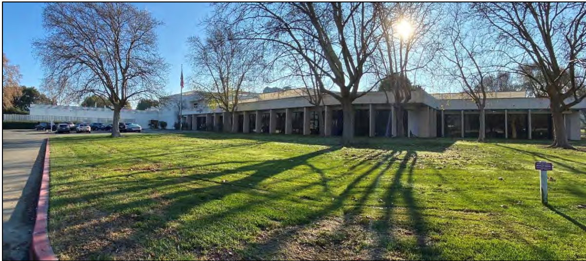
Photograph 3: North side of building complex, with two-story building hyphen on left, facing southeast, December 16, 2022.
