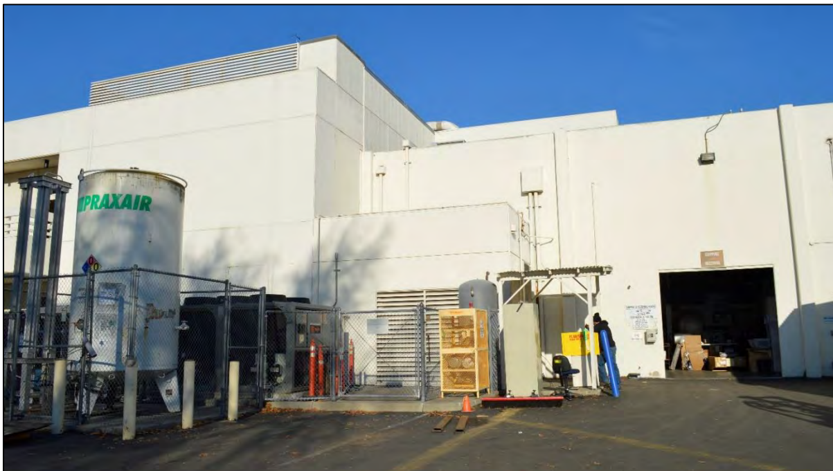
Photograph 8: Two-story office section (on left) and overhead entry door into laboratory section (on right) on south side, facing north, December 16, 2022.
