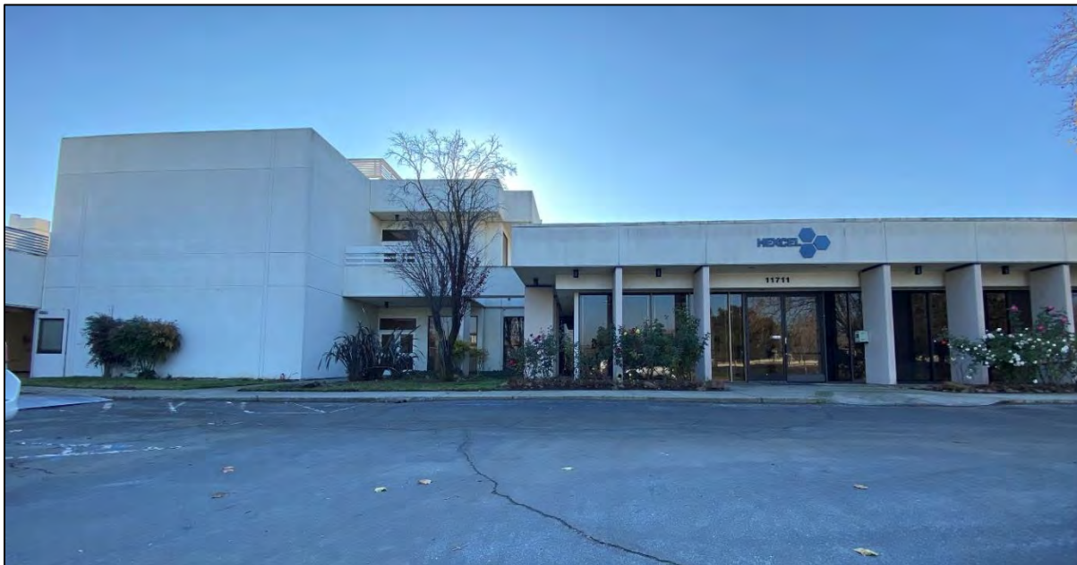
Photograph 4: Detail of north side of the building complex with two-story hyphen on left. Note the recessed window near the center of the frame faces an interior courtyard (see Photographs 15 and 16), facing south, December 16, 2022.
