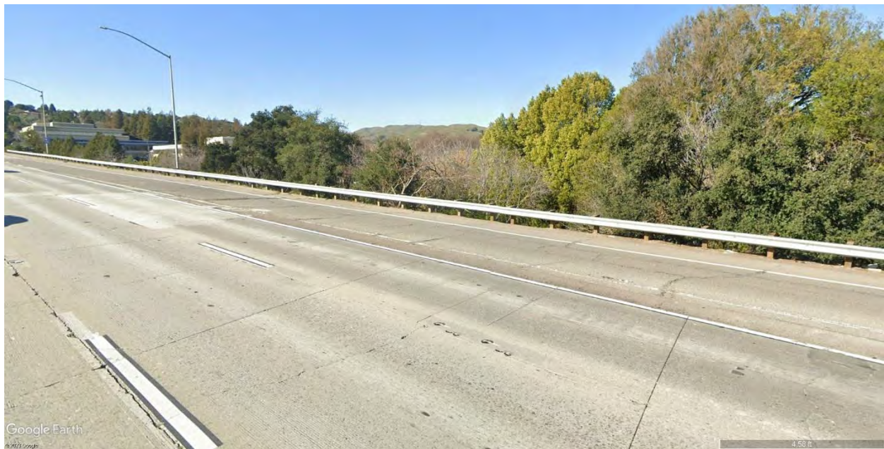
Photo 3: View of the Project site by Motorists Traveling Westbound on I-580
