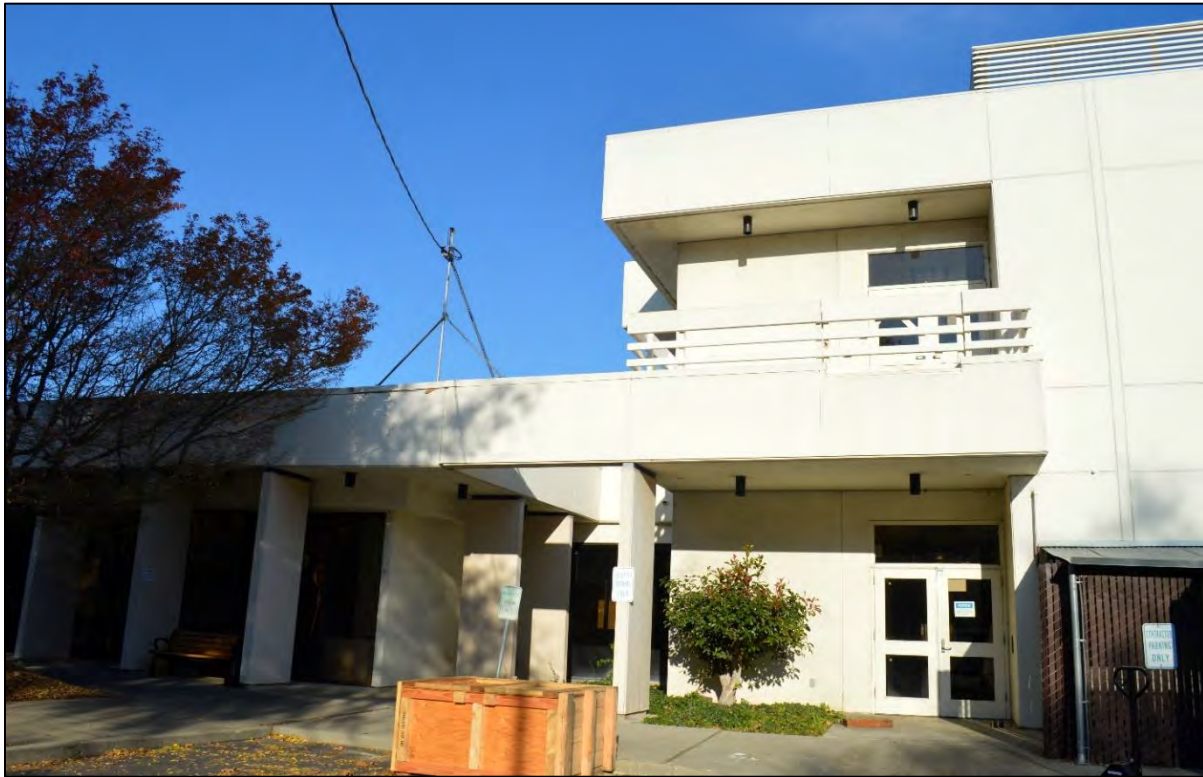
Photograph 7: Detail of entrances in two-story building hyphen on south side, facing north. Note the window at the center of the frame faces an interior courtyard (see Photograph 16).
