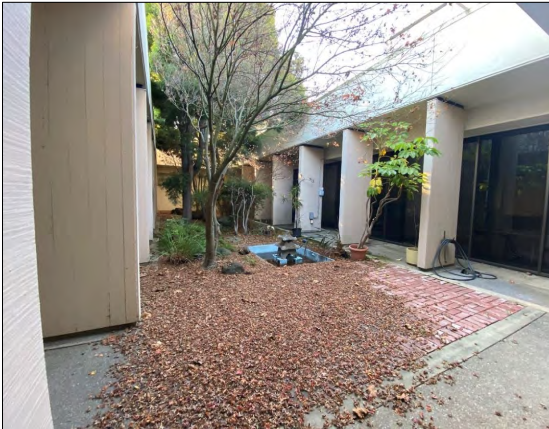
Photograph 18: Overview of west courtyard, facing southwest, December 16, 2022.
