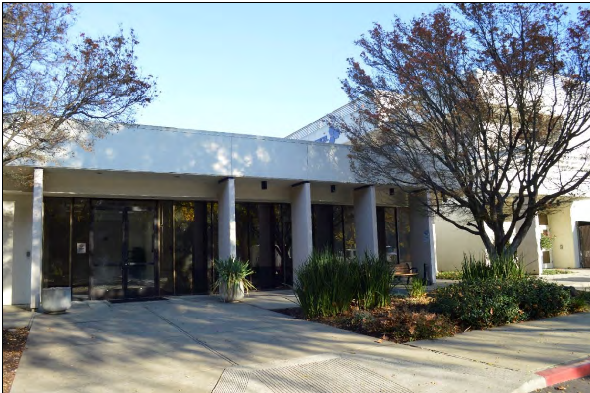
Photograph 6: Detail of entry on south side, facing north, December 16, 2022.
