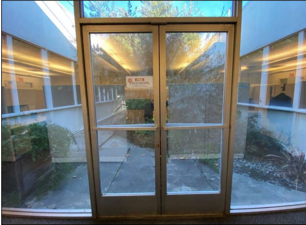
Photograph 13: Southern entry into the east courtyard, facing north, December 16, 2022.
