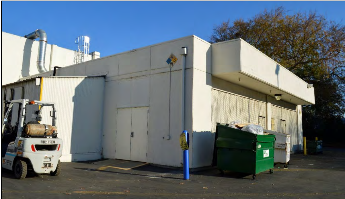
Photograph 9: Southeast corner of building complex, facing northeast, December 16, 2022. Note this section was added in 1985.
