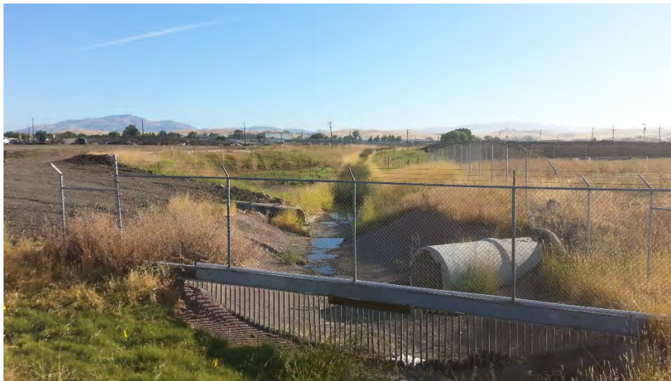
Photo 2: Overview of Chabot Canal and multiple culverts, viewing northeast.
