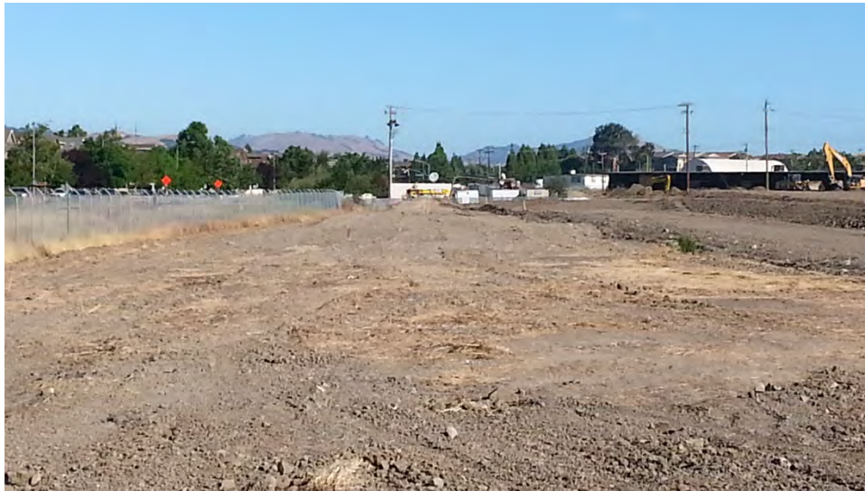
Photo 4: Overview of survey area north of Dublin Blvd, viewing northwest.
