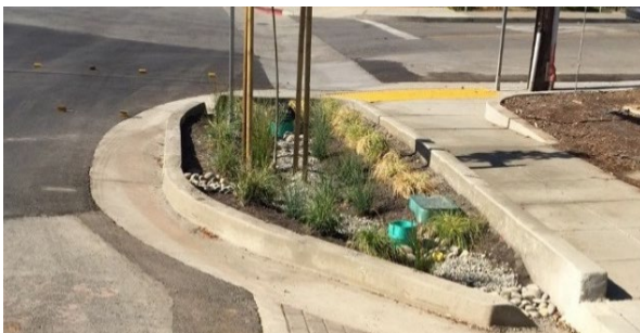
Bioretention Curb Extension in Union City
