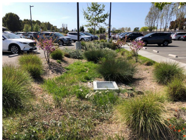
Bioretention Area in the City of Alameda
