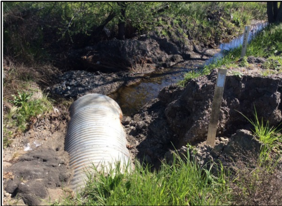
Photo 4. Culvert outlet emptying into the perennial stream (unnamed tributary) that runs parallel to Croak Road and parcel A.
