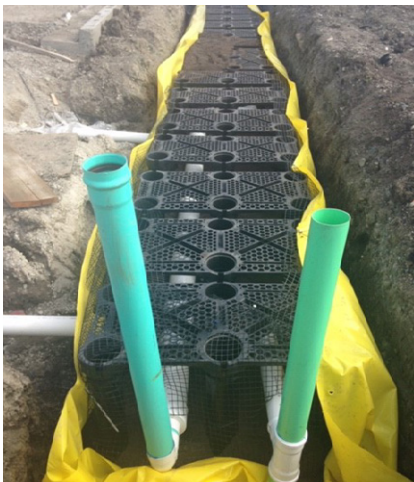
Tree well filter being constructed using Silva Cells at the Boulevard.
