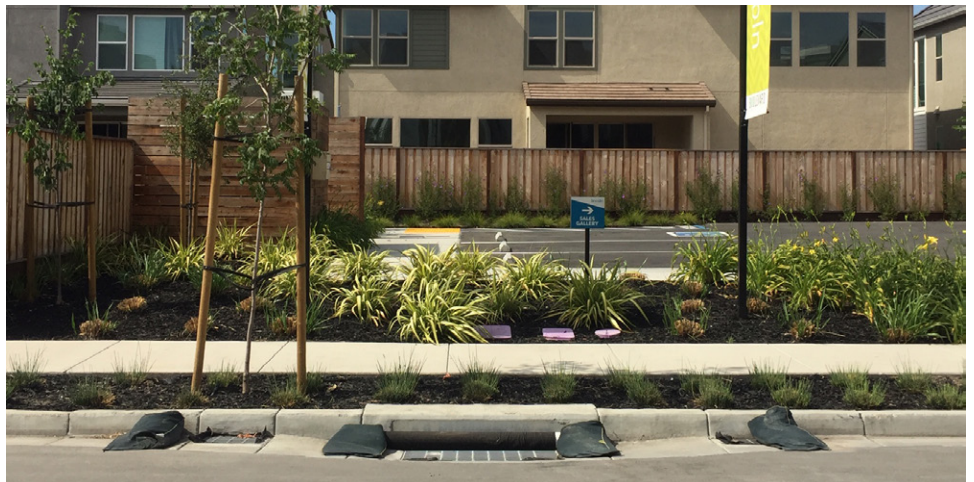
Installed tree well filter using Silva Cells at the Boulevard.
