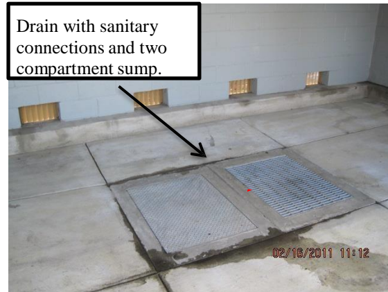
Figure 8: Sanitary connection with sump
